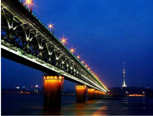
First Yangtze River Bridge, Wuhan
